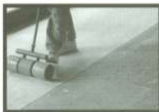
Embed SIS with a roller
