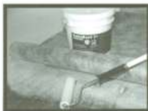
Apply bonding agent (either NobleBond 21 adhesive or latex modified thin-set)
