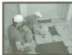
Install tile by a thin-bed method
